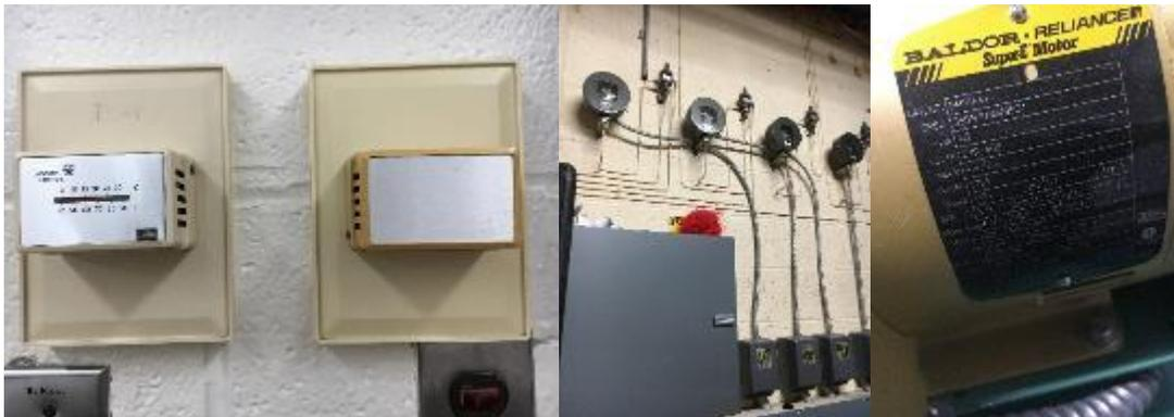
*Figure 11-Pneumatic Control System*
