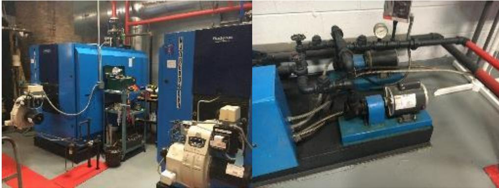
*Figure 8-Boilers and Hot Water Heating System*
