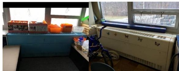
**Figure 12- Unit Ventilators**
