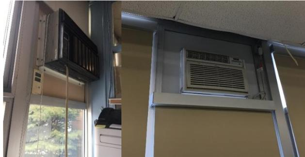
*Figure 13-Typical Window AC Units*
