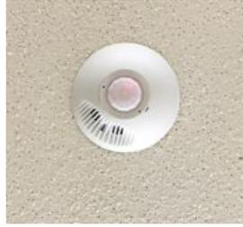
**Figure 9- Typical Remote Mounted Lighting Occupancy Sensor**
