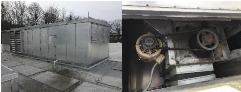
*Figure 11 - Package DX Cooling*
